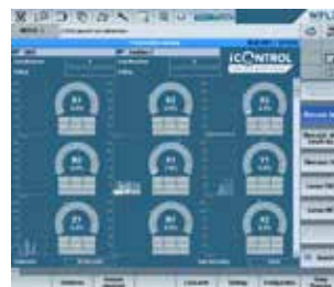
Surveillance du process (iControl)
